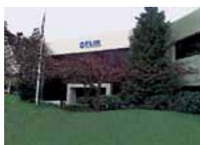
FLIR Systems, Portland
